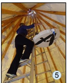
Untie the black tape from the strings and use the carabiner to hook the Rain Catcher to the tripod rope or an eye screw that you screw into the pole cluster. The Rain Catcher strings will tilt the pan towards the spout where the water will drip out (4).
